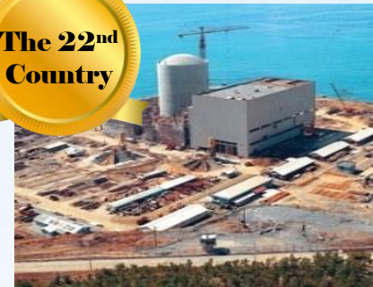
Construction of Kori-1(587MWe)** (1971~1978)
